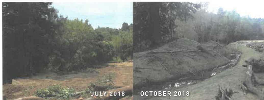
In just a few short months, the Tocaloma project area (pictured on the left in late July) has become a water-receiving side channel, providing shelter and sustenance for young salmonids.
